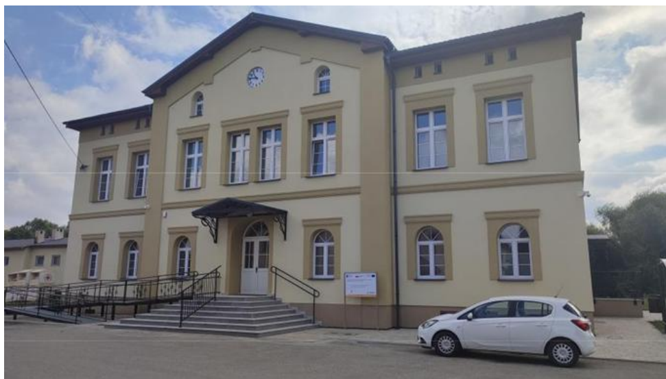
Figure 18 Community Services Centre building in Pietrowice Wielkie, photograph.
