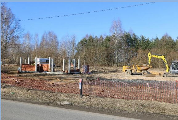
Construction of a transfer hub in Psary, source: Psary municipality
