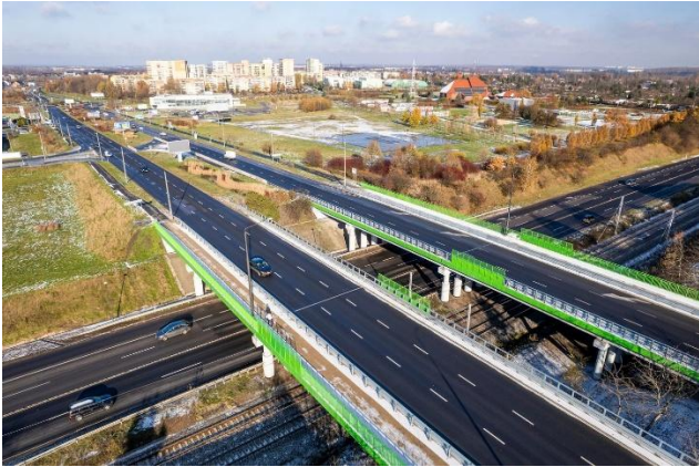
Flyover over national road DK 88 in Zabrze, source: Zabrze City Hall website
