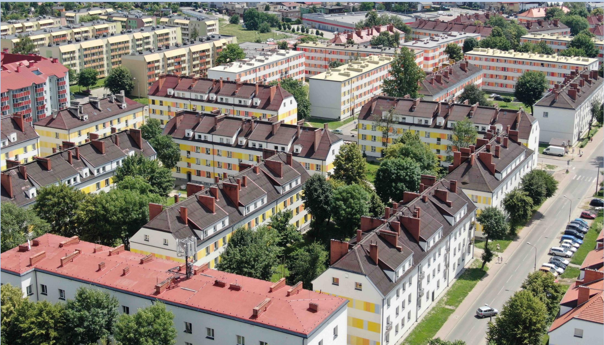
Connecting buildings to district heating sources and thermal modernisation in Piekary Śląskie, source: Town Hall in Piekary Śląskie
