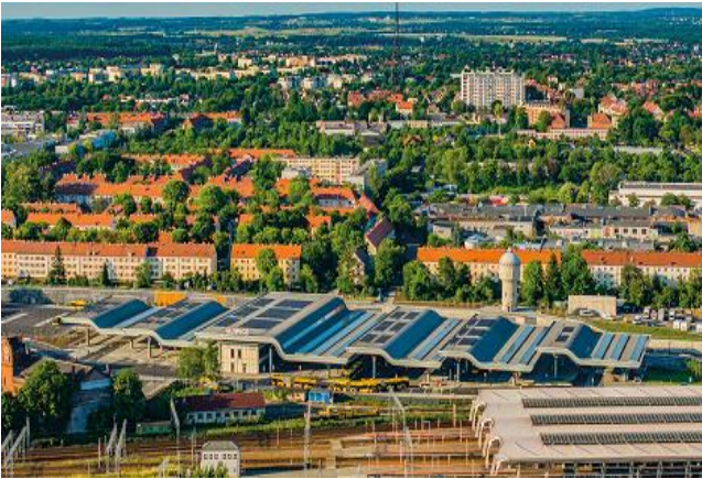
Transfer Hub in Gliwice, source: Gliwice City Hall
