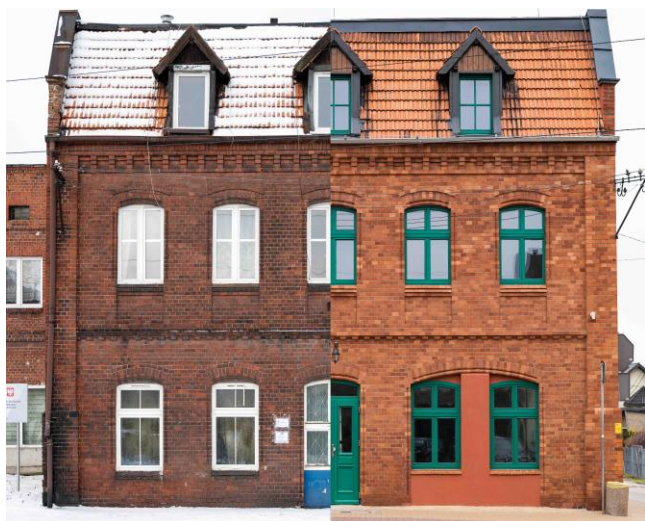
Thermal modernisation of a historic building in Tychy, source: Municipal Residential Building Management Authority in Tychy
