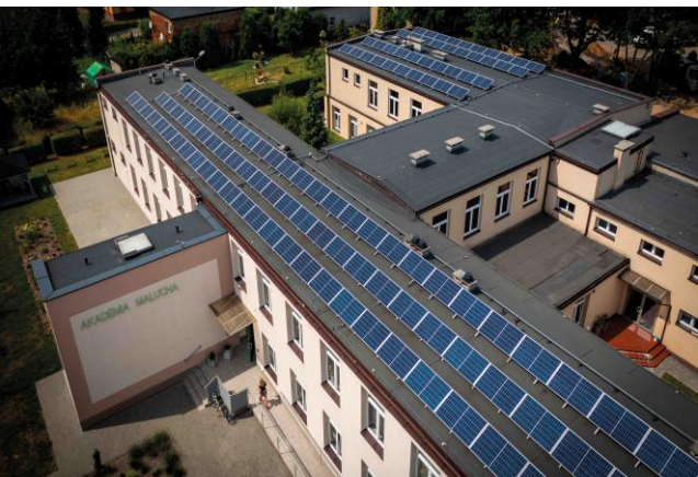
Photovoltaic installation in Świerklaniec, source: Świerklaniec Municipal Office
